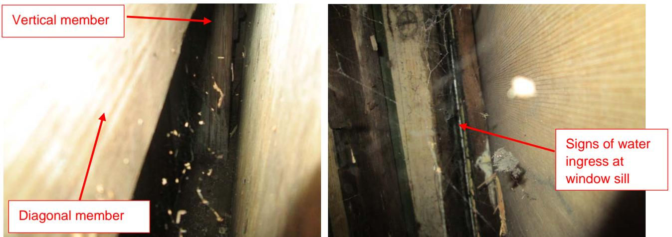
Figure 7: View towards Platform 1 and a view looking up to the window sill in Panel 5
