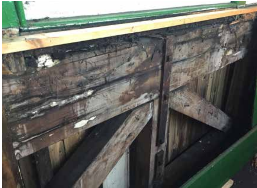
The bridge frame exposed during the inspection
