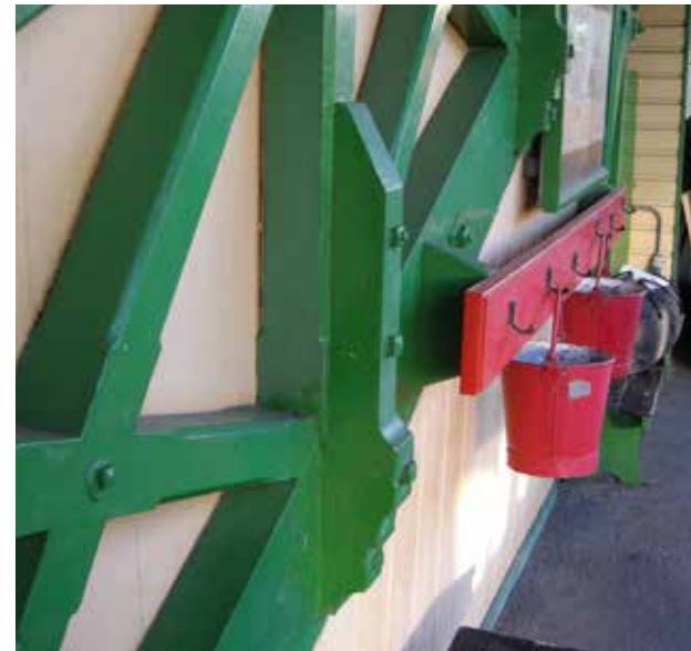
The shaped wooden brackets, platform 3
